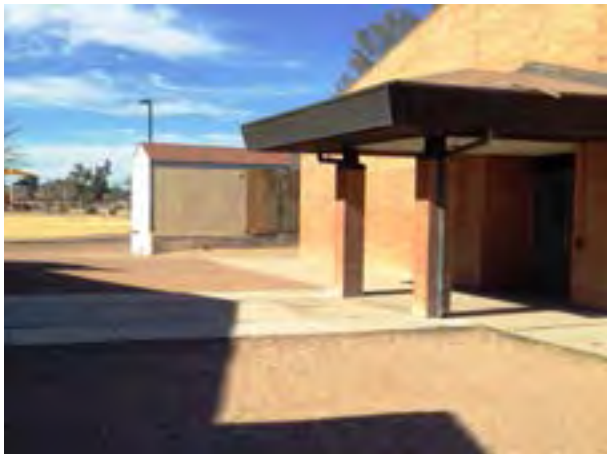
Boarded up portable bathrooms at Grijalva Elementary
